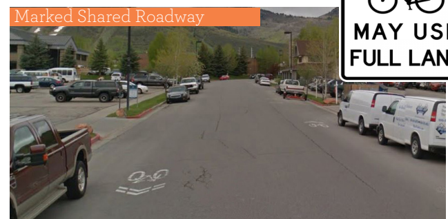
Marked shared roadway on Prospector Ave.
