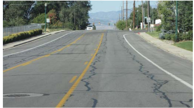
Wide roadway on E. 1600 North near N. 500 East
