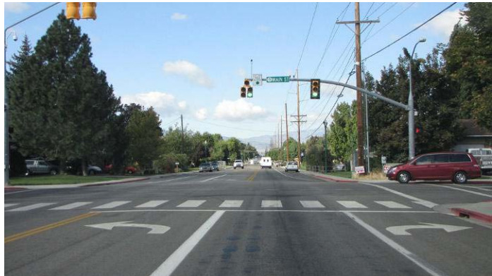
'Transverse' and 'piano key' crosswalk striping near North Ridge Elementary School at 1600 North and Main Street
