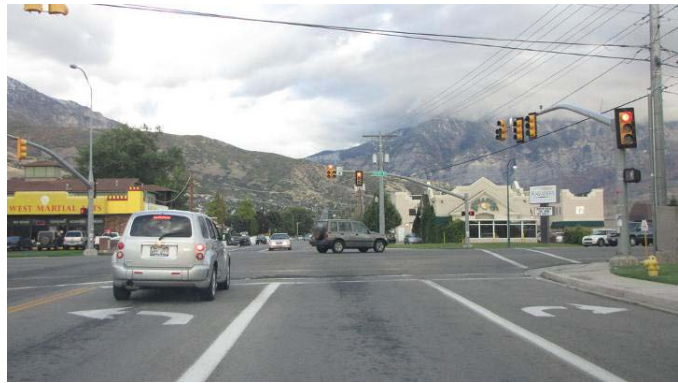
Transverse crosswalk markings at 2000 North at State Street
