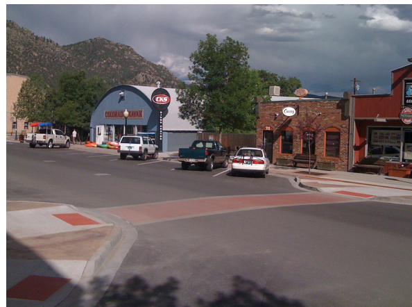
Curb extensions shorten crossing distances for pedestrians and can calm traffic as well
