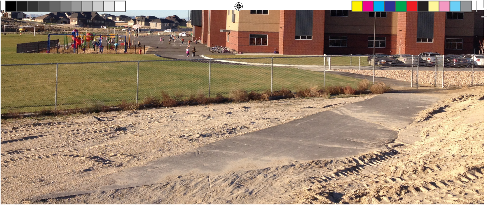
Dirt from adjacent development on a shared-use path leading to Black Ridge Elementary
