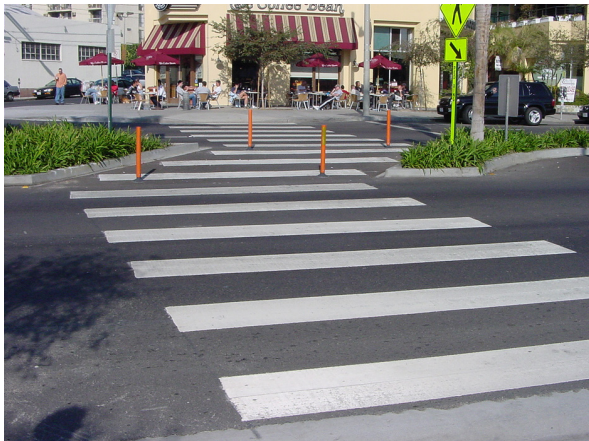
Median refuge island
