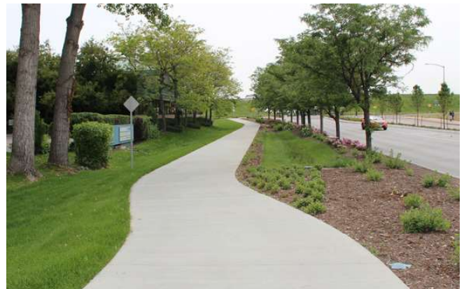
Concrete shared use path
