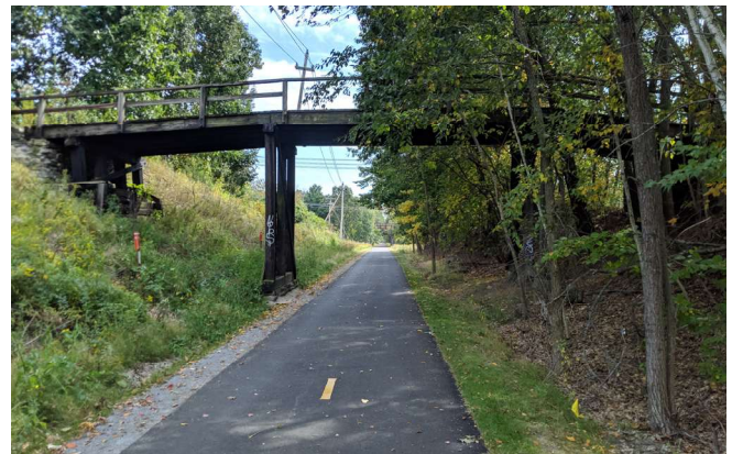
Rail to trail undercrossing
