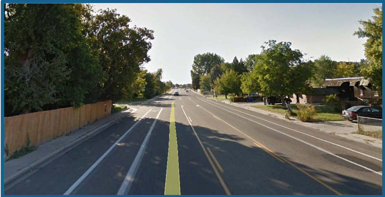
Figure 22. View of 820 North looking west at approximately 1300 West.
